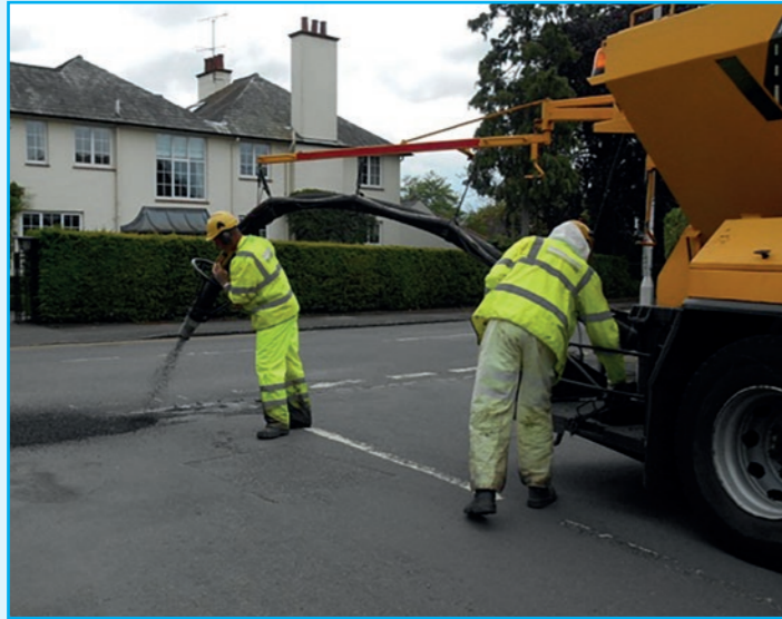
This Jetpatcher, seen in Bulstrode Way, repairs 10 to 15 holes an hour. The vehicle has a driver, a patcher, his assistant, and a traffic manager.
